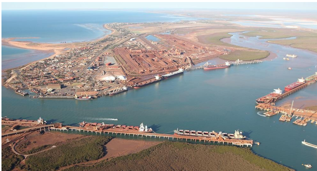
Image: Port Hedland Iron Ore Export Facilities
